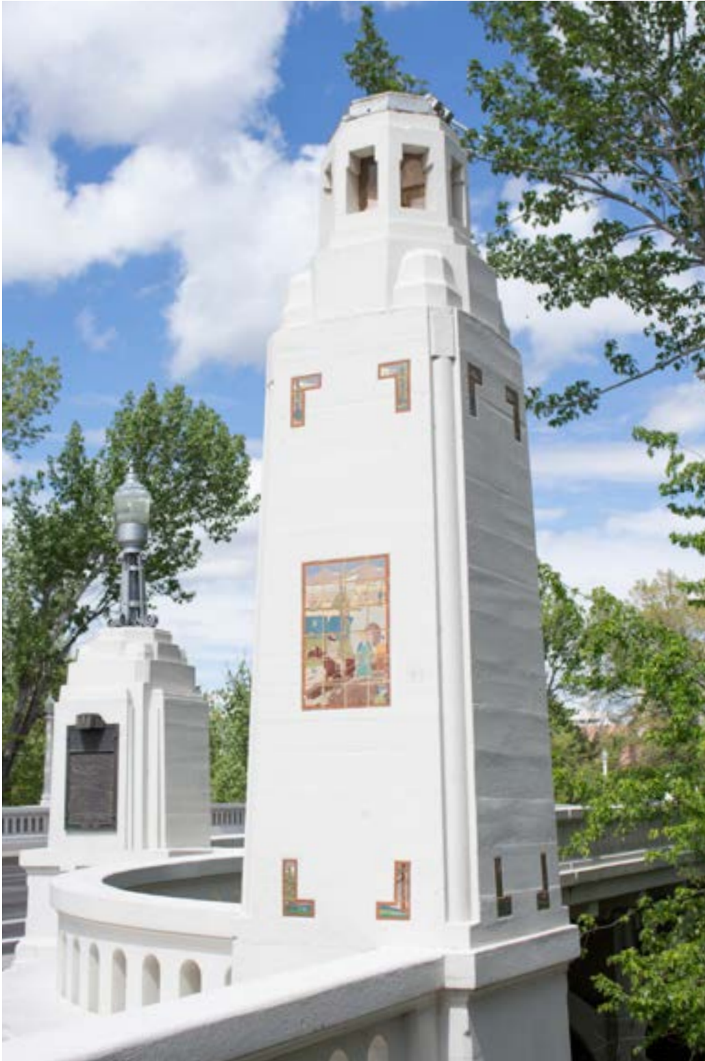
Oregon Trail Memorial Bridge
